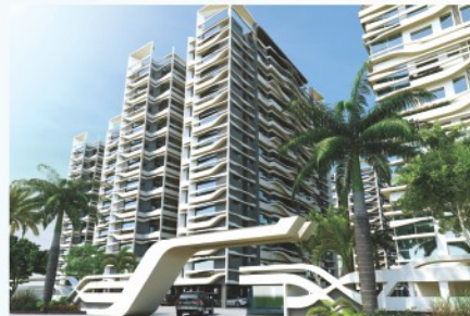
Automatic Entry Gate
